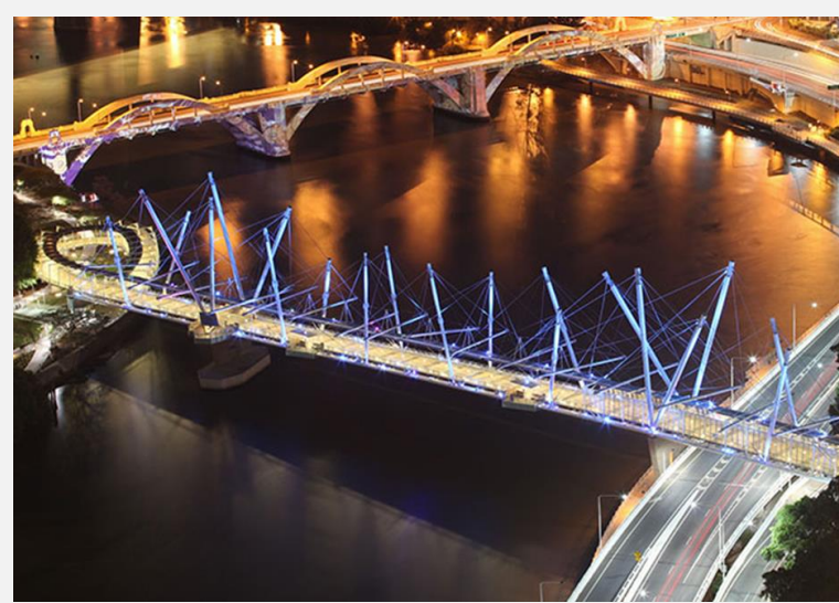
Kurilpa Bridge in Brisbane in Tensegrity-Bauweise
